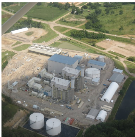
AEP's Dresden gas plant in Ohio Source: AEP
